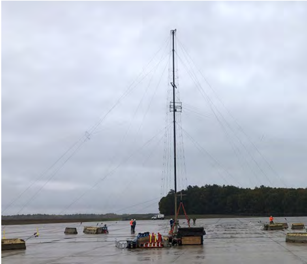
Figure 2-2. Photograph of a Mobile CWMS Antenna (typical)
